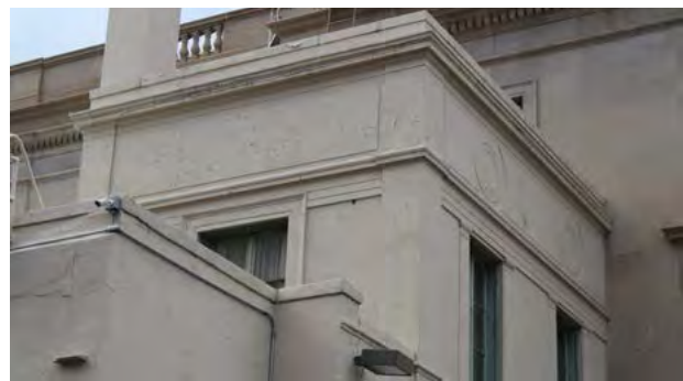
Figure 027 Detail of stucco cladding. EHT Tracerics.
