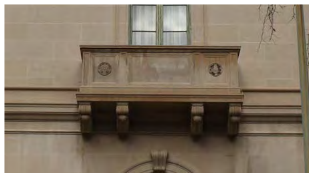
Figure 024 Projecting balcony on north elevation. EHT Traceries.
