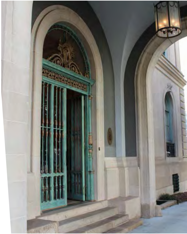
Figure 035 Main entrance door and ornamental grille. EHT Tracerics.
