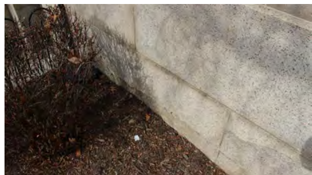
Figure 026 Detail of granite water table. EHT Tracerics.
