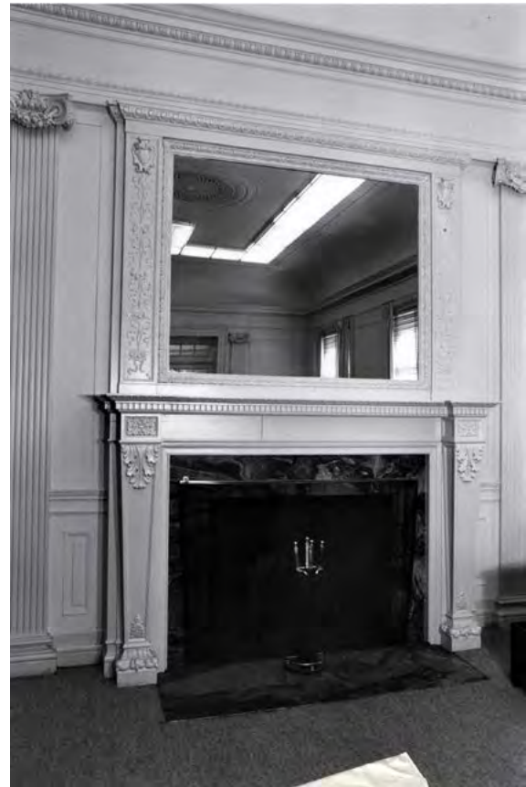
Figure 013 Detail of Dining Room fireplace, 1973. Note the uniform color scheme, carpeted floor, and surface-mounted fluorescent light reflected in the overmantel mirror. U.S. Commission of Fine Arts, Vertical Files.
