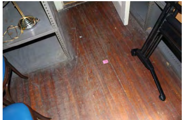
Figure 045 Original wood plank floor on basement floor. EHT Traceries.
