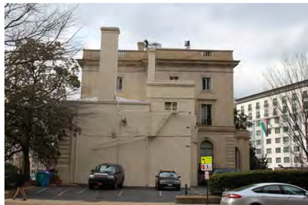
Figure 021 Variety of chimneys visible on east elevation. EHT Tracerics.
