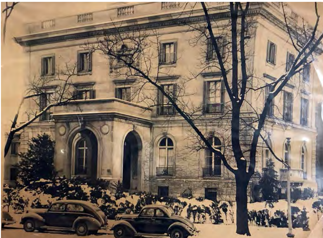
Figure 032 Original window configuration and details on the north elevation, 1940. Evening Star , Washingtoniana Collection, DC Public Library's Special Collections.
