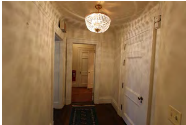
Figure 073 Corridor east of Entrance Hall. EHT Traceries.
