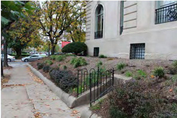
Figure 039 Planted berm, curb, and vault along southern edge of site, facing west. EHT Traceries.
