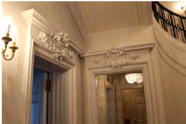
Figure 054 Detail of door surrounds and overdoor architraves. EHT Traceries.
