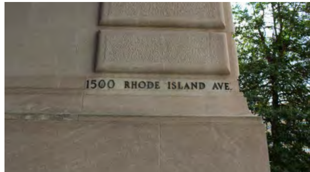
Figure 025 Detail of honed and tooled limestone finishes on north elevation. EHT Tracerics.
