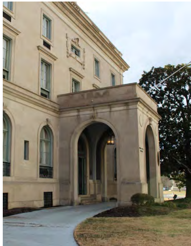
Figure 023 One-story porte cochère projection on the north elevation. EHT Traceries.
