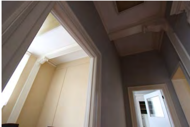
Figure 078 Original bulkhead feature spanning across partition walls. EHT Tracerics.
