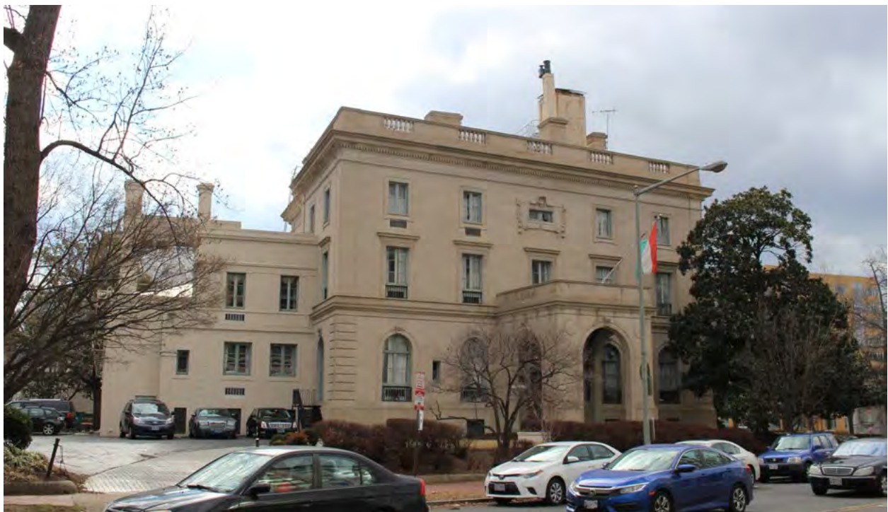
Figure 018 North elevation, facing southwest. The building's three-story, primary volume is juxtaposed against a lower extension to the east. EHT Tracerics.
