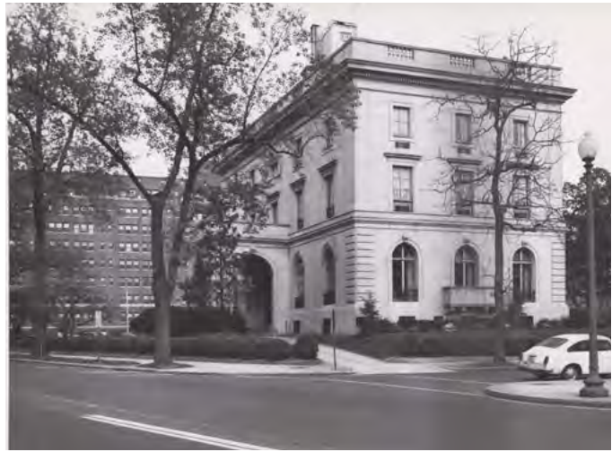
Figure 015 North and west elevations, showing new exterior vents beneath window openings, 1970. U.S. Commission of Fine Arts, Vertical Files.
