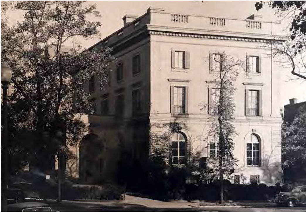
Figure 031 Detail of original window configuration and details on the north and west elevations, 1940. Evening Star , Washingtoniana Collection, DC Public Library's Special Collections.
