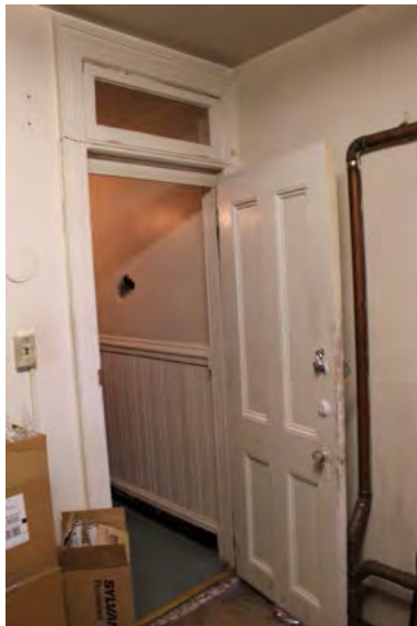
Figure 049 Original door, transom, and surround on basement floor. EHT Traceries.
