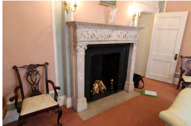
Figure 064 Detail of Office fireplace. EHT Tracerics.
