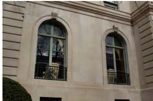
Figure 034 Balconette window railings on first story. EHT Tracerics.
